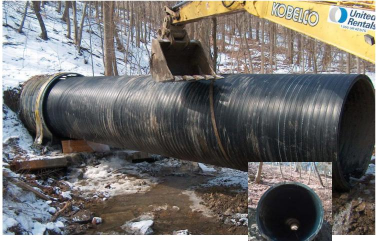
The residents of the village of Gates Mills, a guiet community just outside of Cleveland, were spared months of traffic and village disruption when Weholite was selected for their culvert rehabilitation project. The existing 120" CMP culvert was under 35' of cover and corroding badly.
